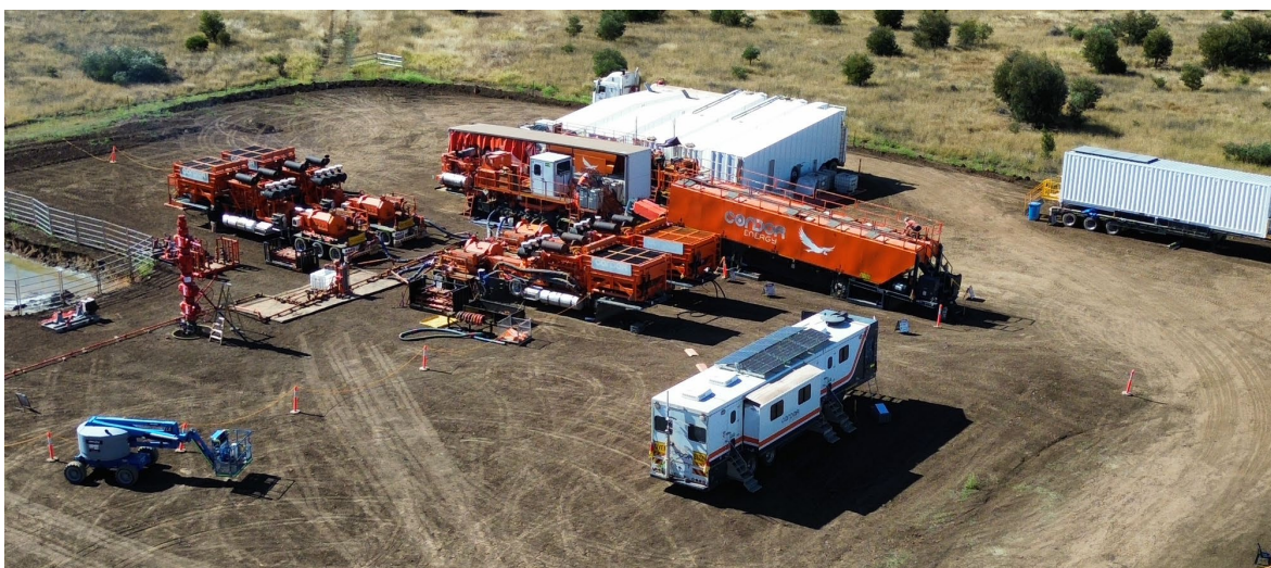
Picture 1: Completions activity on R5 well pad
