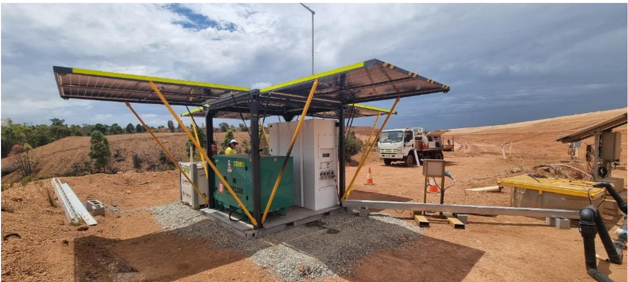
Installation of a new hybrid power unit in Western Australia
