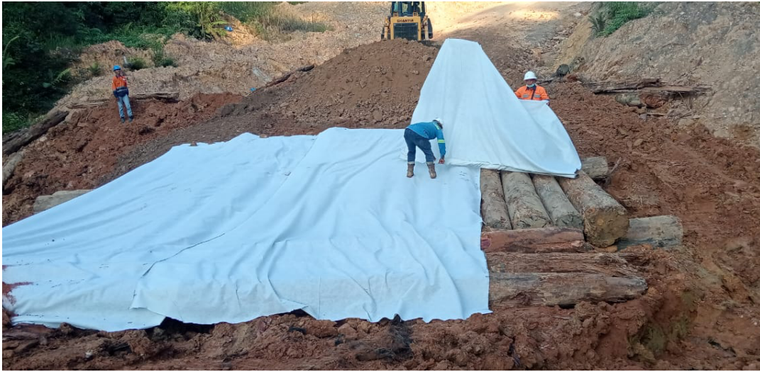
Bridge repairment at km 90
