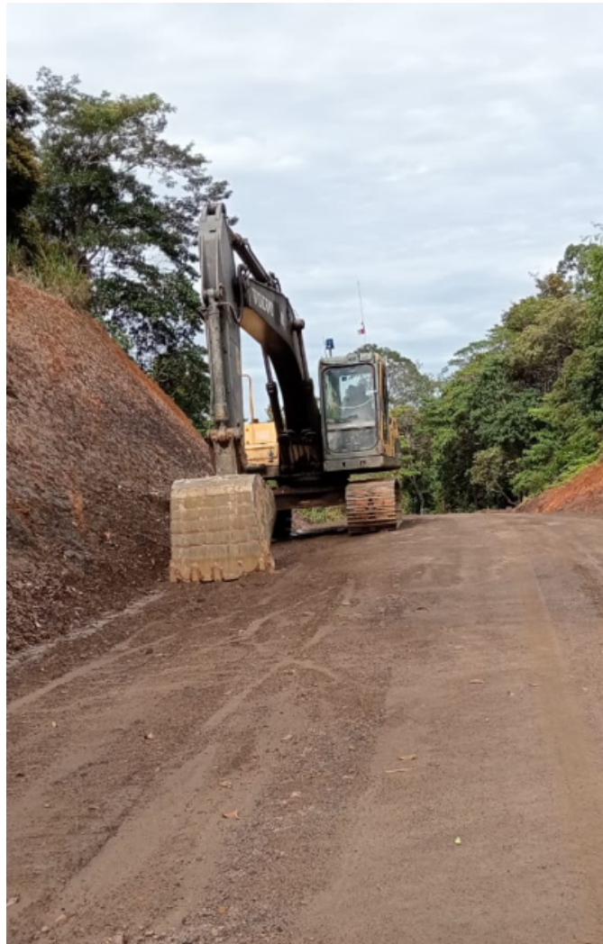
Road maintenance km 93
