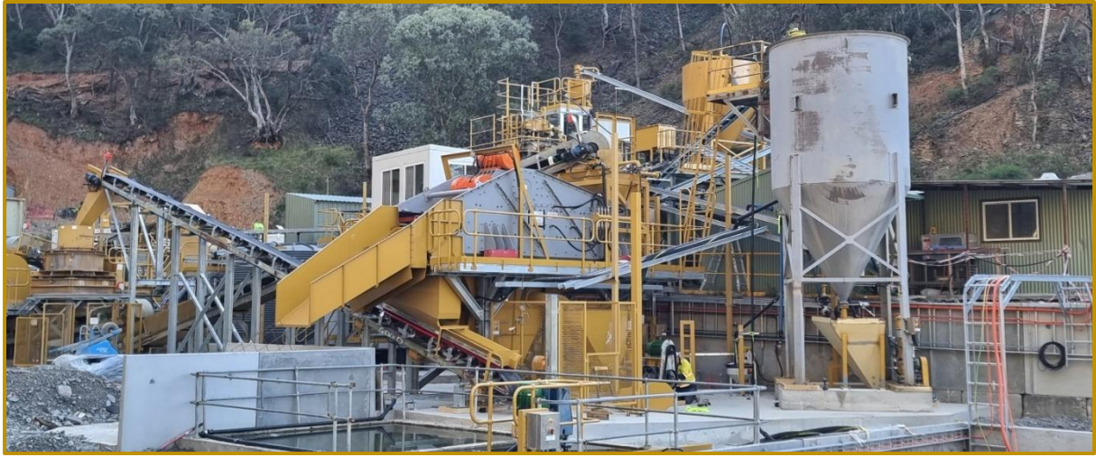
Figure 16: Reward gold gravity plant looking back over the crushing circuit
