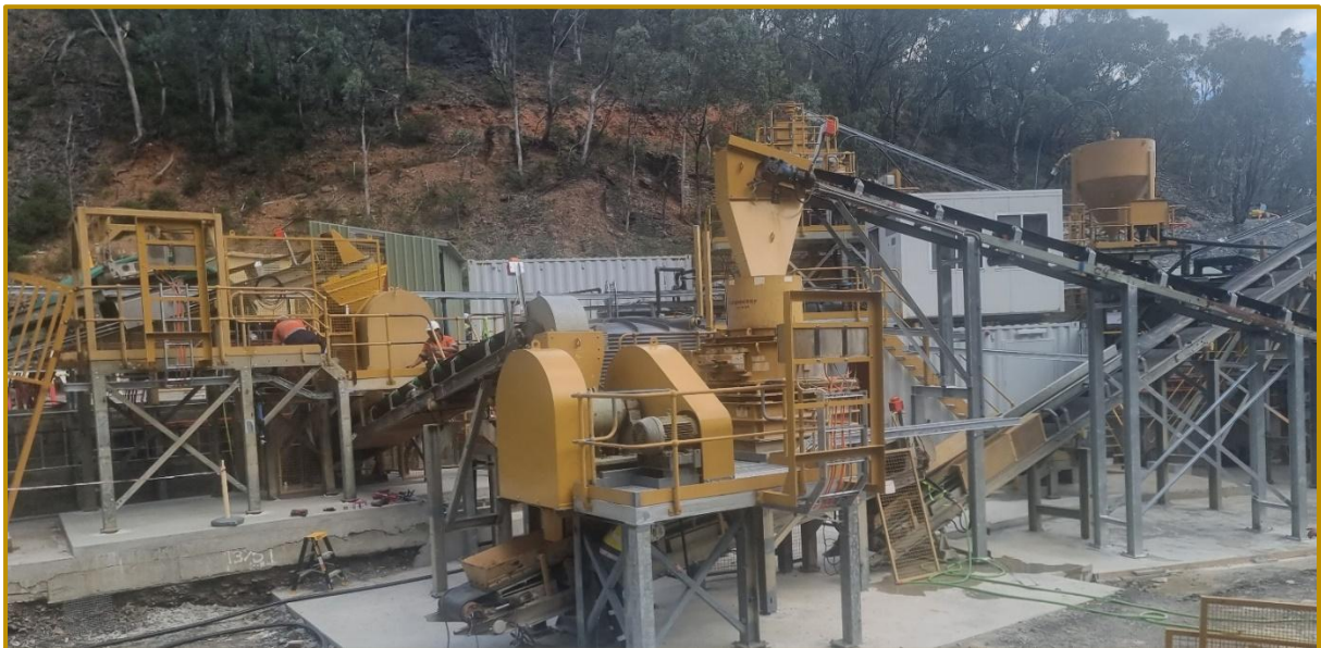
Figure 17: Reward gravity gold plant looking over the 2 jaw crushers and the impact crusher
