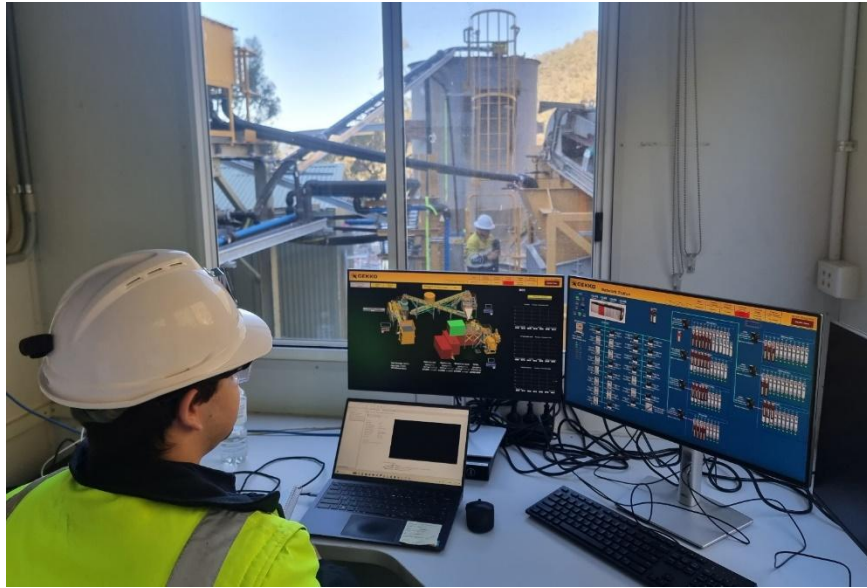
Figure 12: Automation programming technician testing the Reward gravity plant systems from control room
