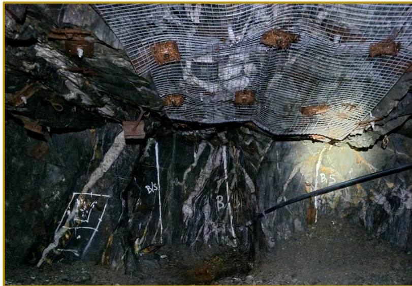
Figure 10 Vertex Technical team have found mine ready stops in the upper workings
