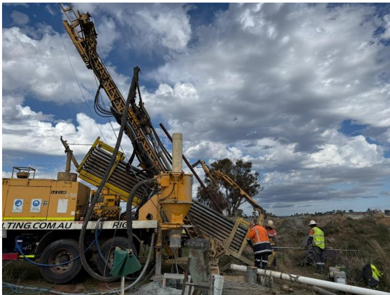
Figure 4: DRILLIT UDR 650 operating at London Victoria Mine
