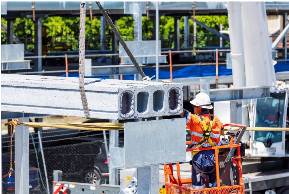
Image 3. Installation of CVB
