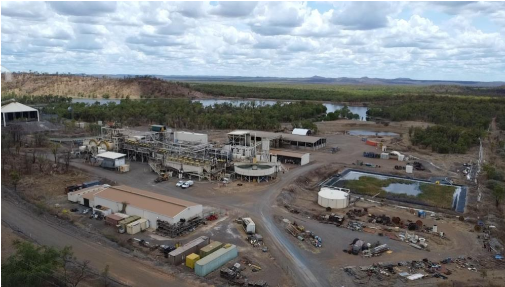
Figure 2. Mungana Processing Plant (Source: Aurora Metals).
