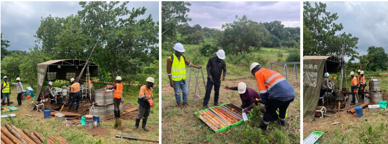
Figure 2: Drilling activities at Didievi
