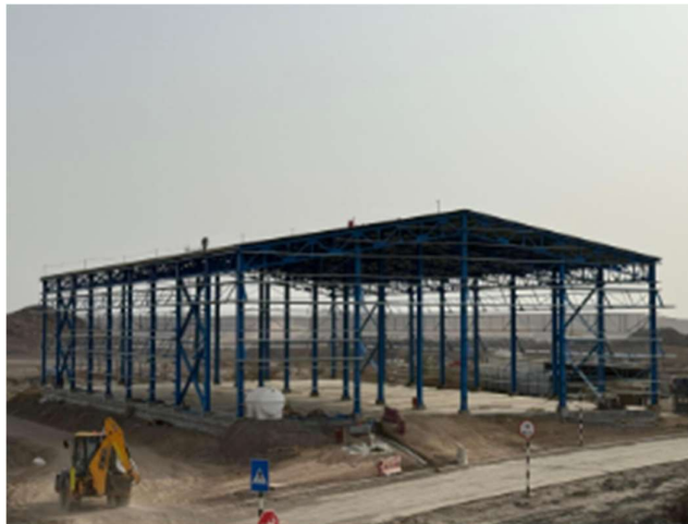
Image: Construction of the new concentrate storage shed
