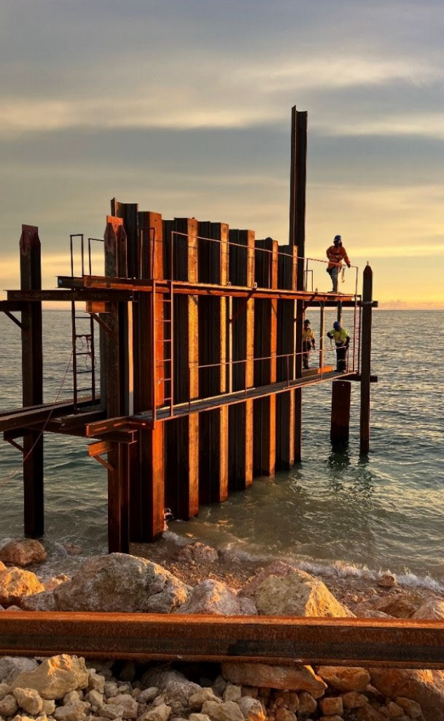
Wharf Sheet Pile Installation
