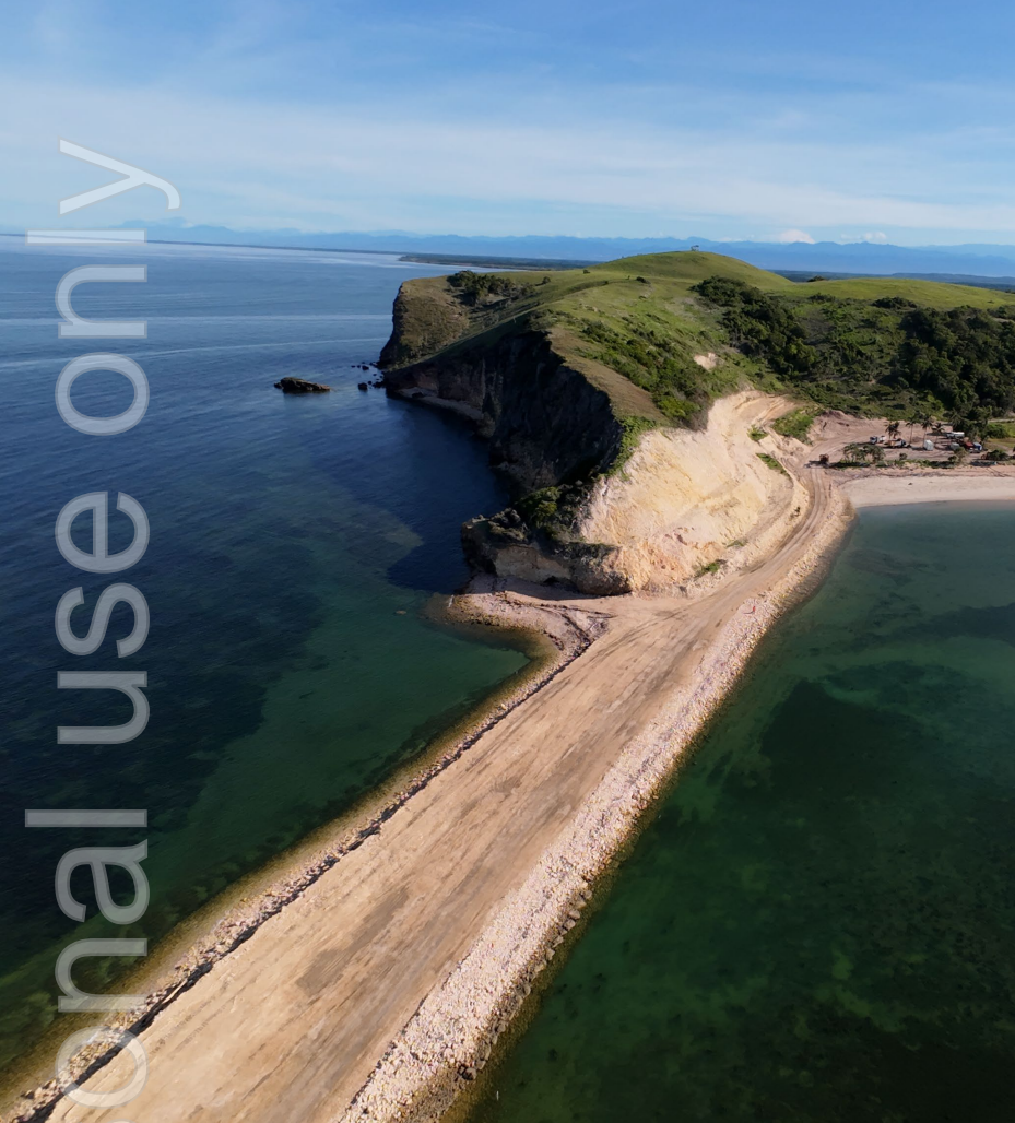
Rubble Wharf Access
