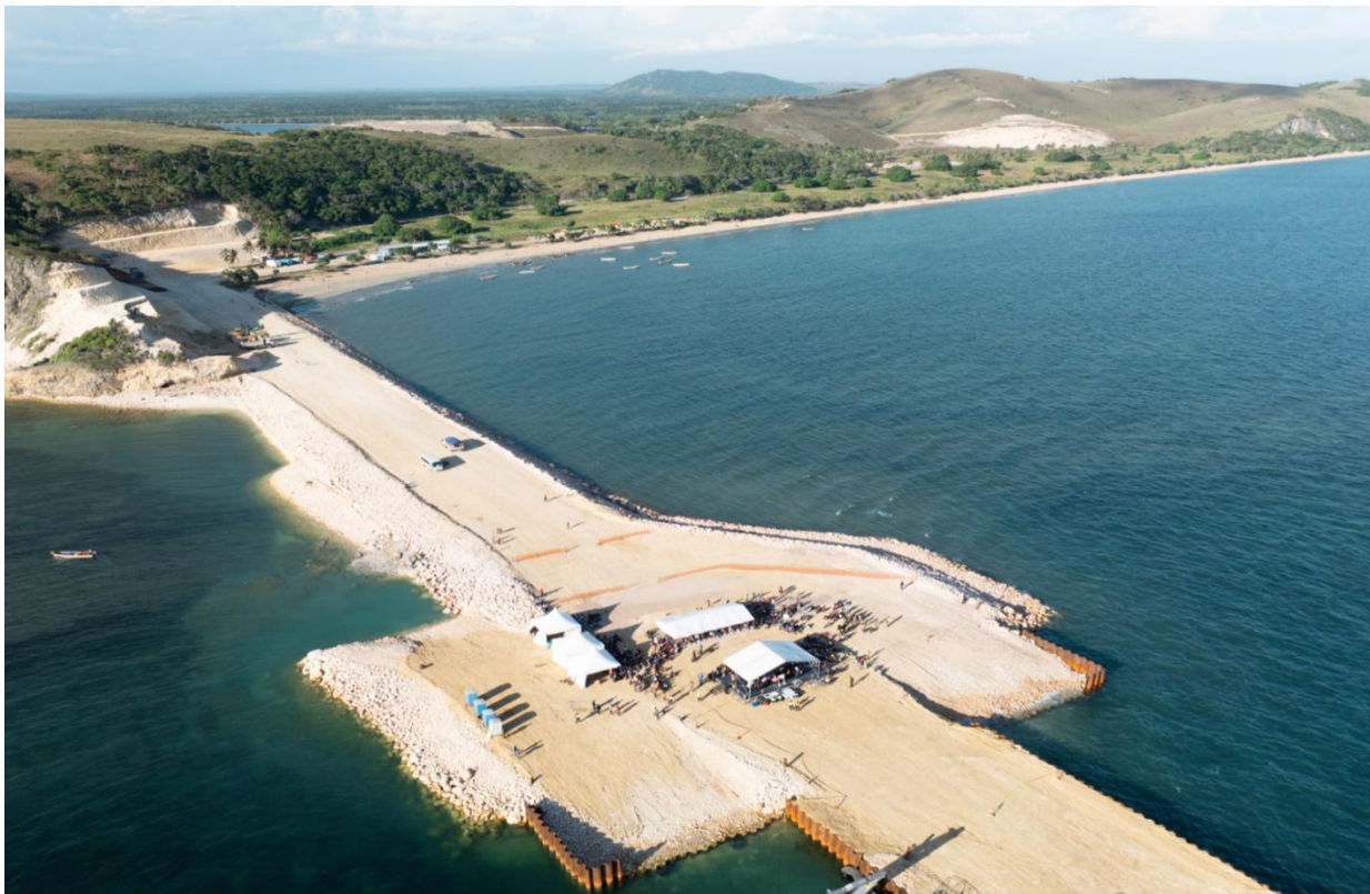
Picture: FID announcement in progress on stage 2 of the wharf.
