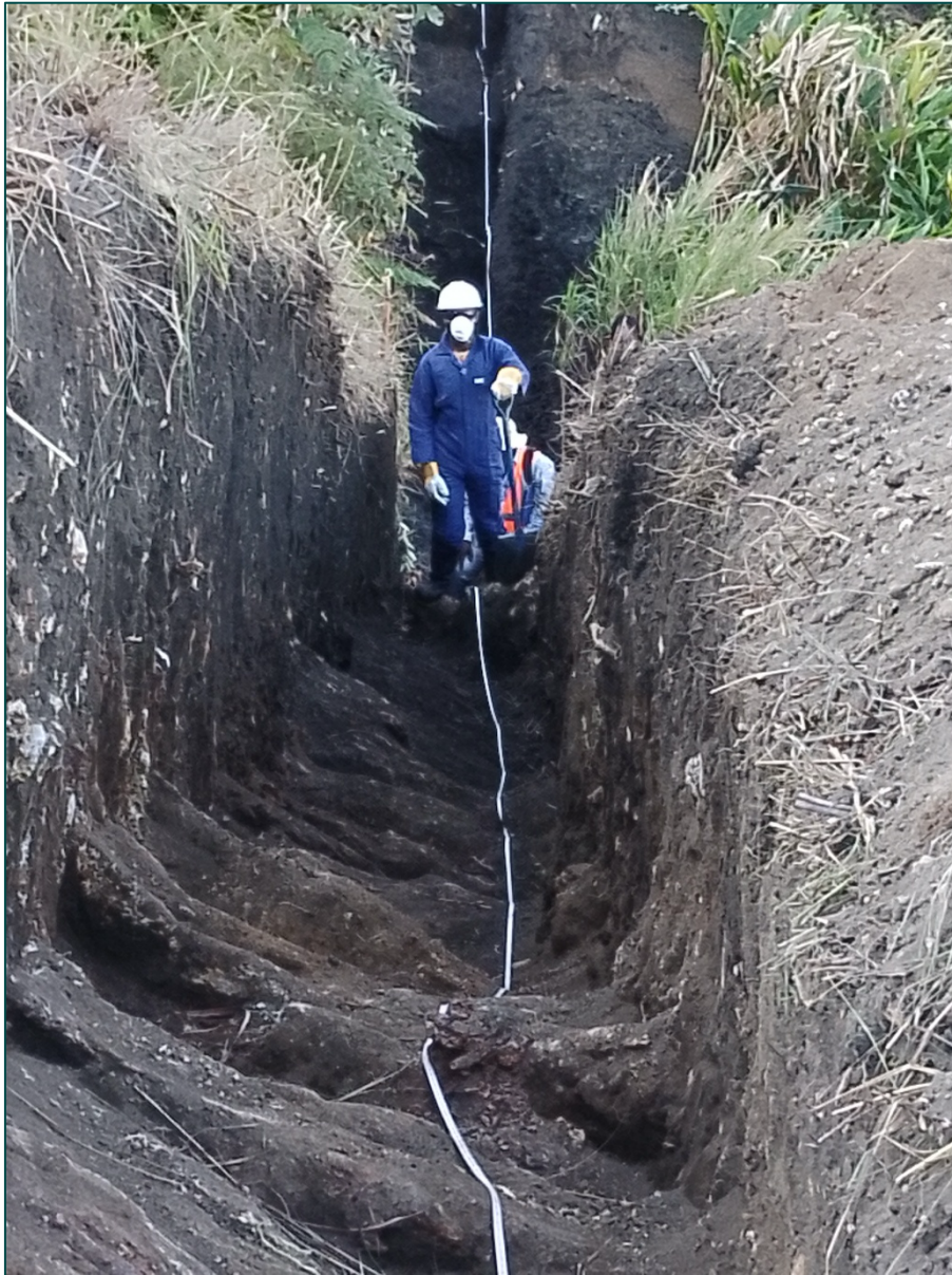
Photo 1: Excavation of trench TRUM23-003.
