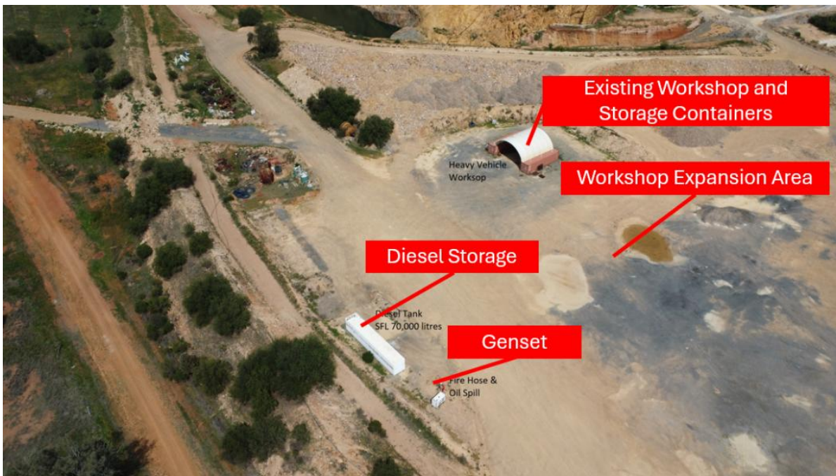
Figure 9: Existing mining and diesel power infrastructure at Mt Boppy
