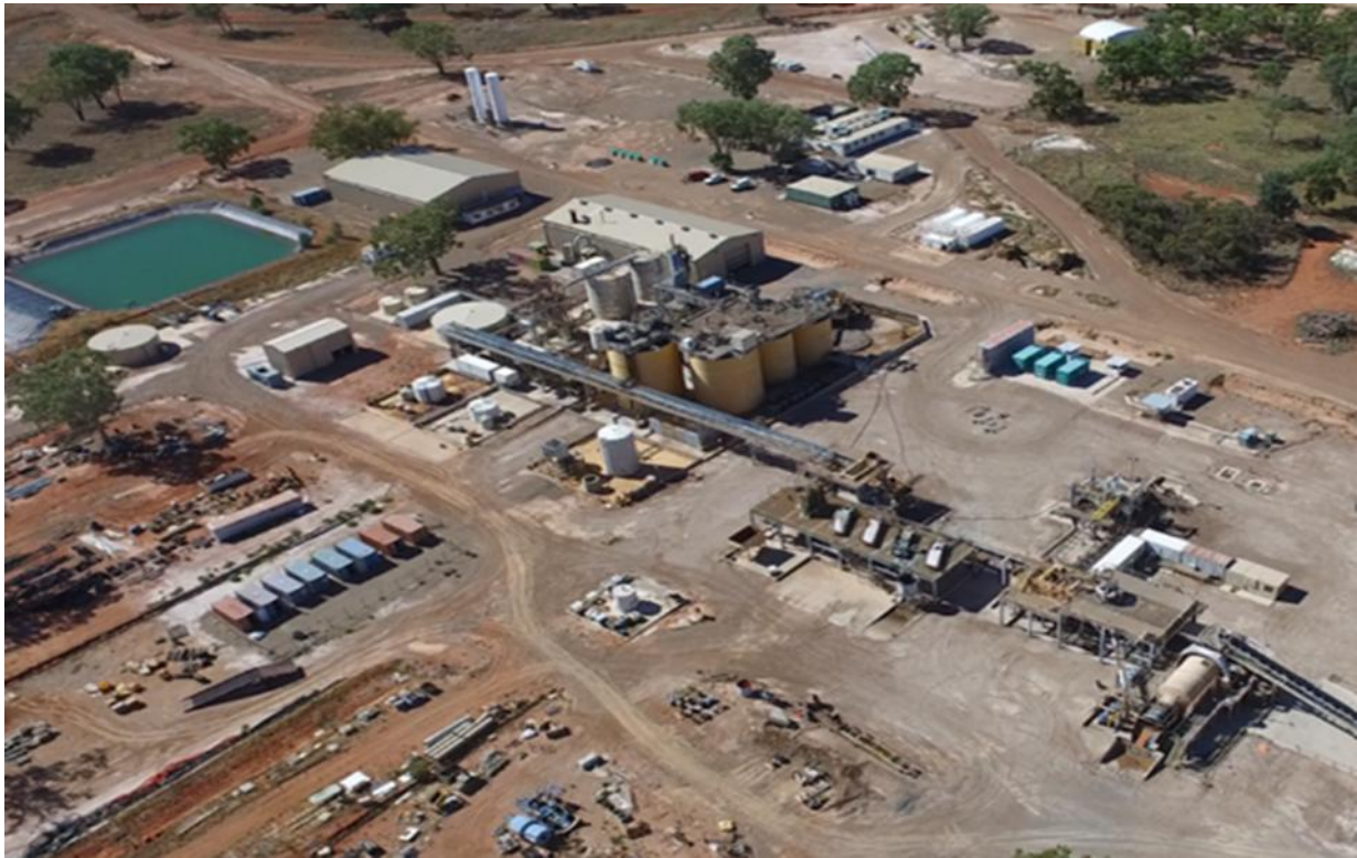
Figure 3: The existing Wonawinta Processing Plant.
