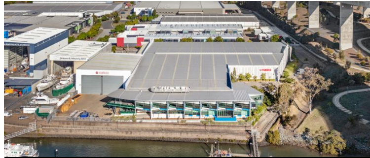
69 RIVERGATE PLACE, MURARRIE QLD 2
