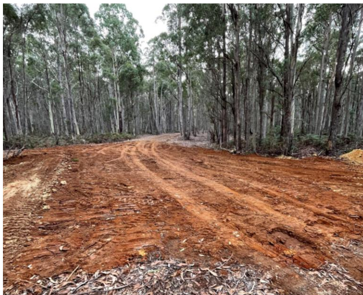
Figure 2: Trial pit area following extraction and rehabilitation of area shown in Figure 1
