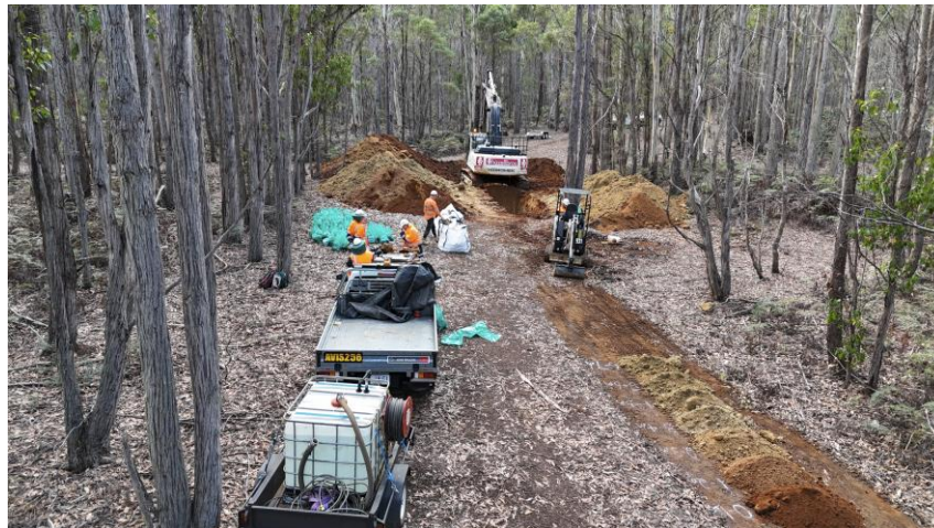
Figure 1: Bulk sample RMP002 being excavated at Deep Leads resource
