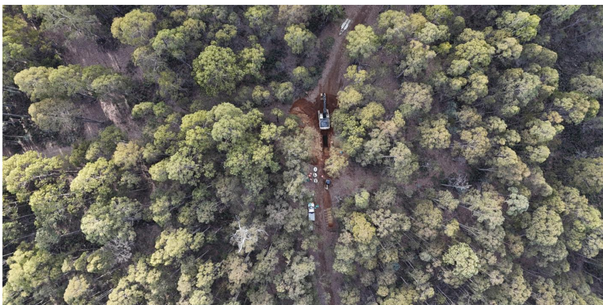
Figure 3: Overhead view of trial pit excavation at Deep Leads
