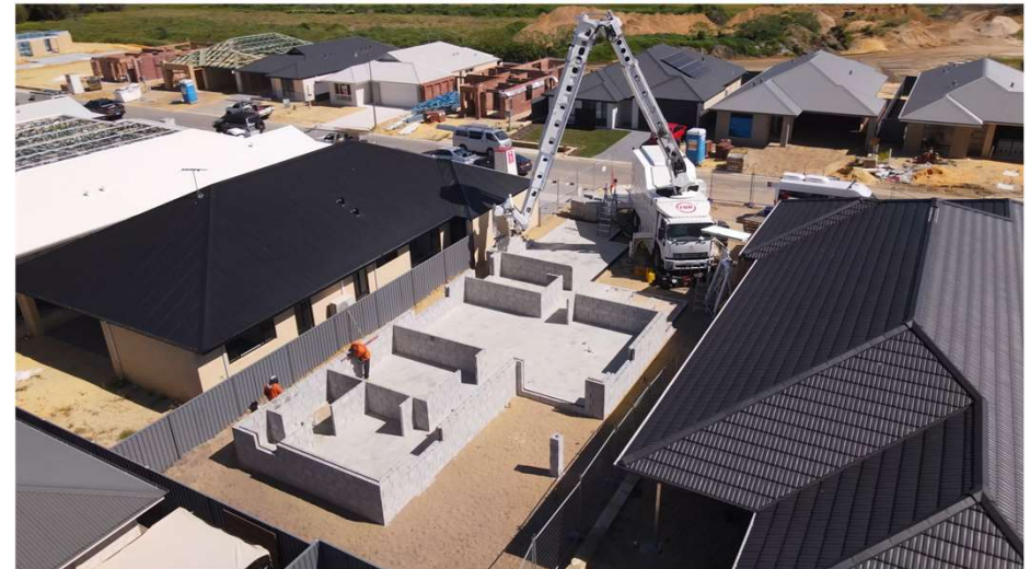
Hadrian X ® building a structure in Perth, generating zero on-site waste
