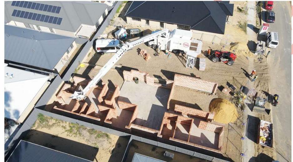
House constructed using Wienerberger Porotherm – world's largest clay blocks
