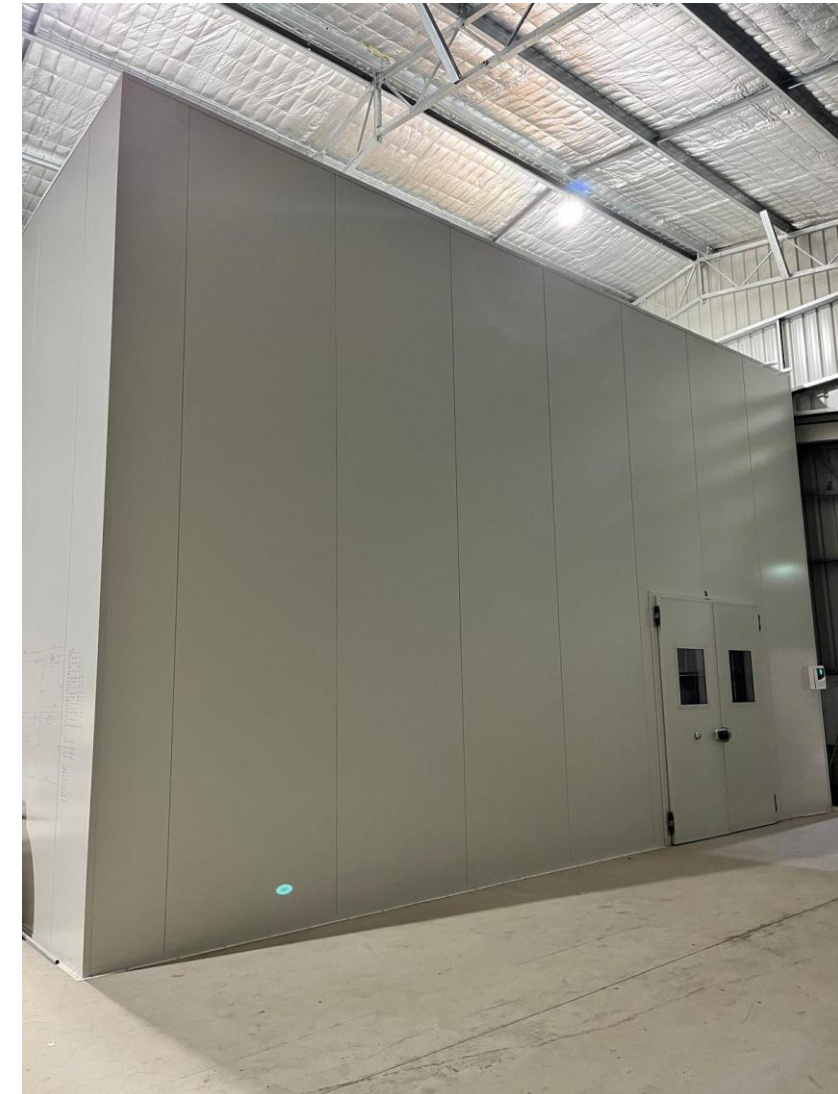
Refrigerated curing room
