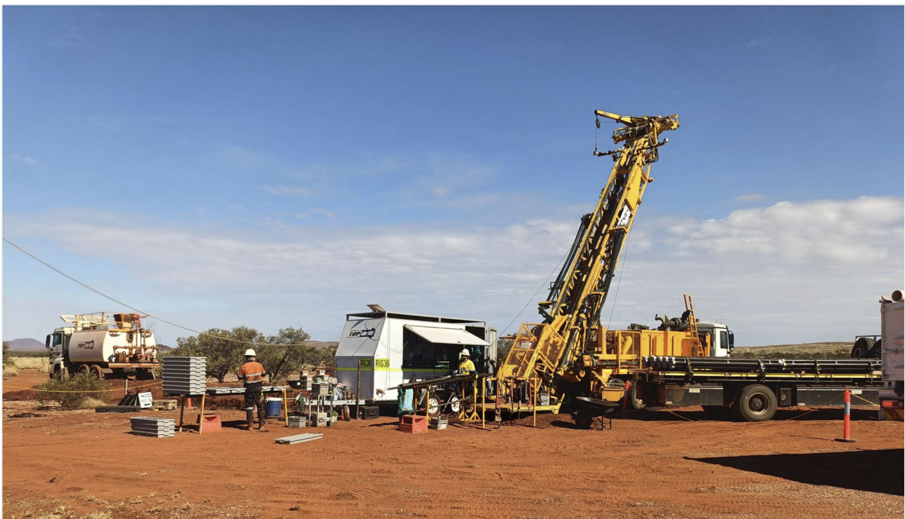
Figure 1: Diamond drilling at the Paulsens West seismic target.
