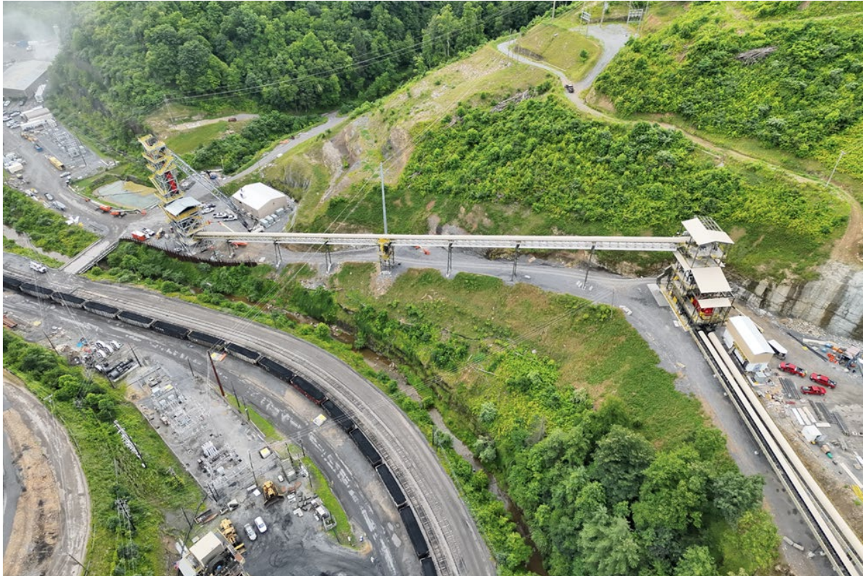
Caption: Buchanan expansion – New Shaft and Surface Infrastructure
