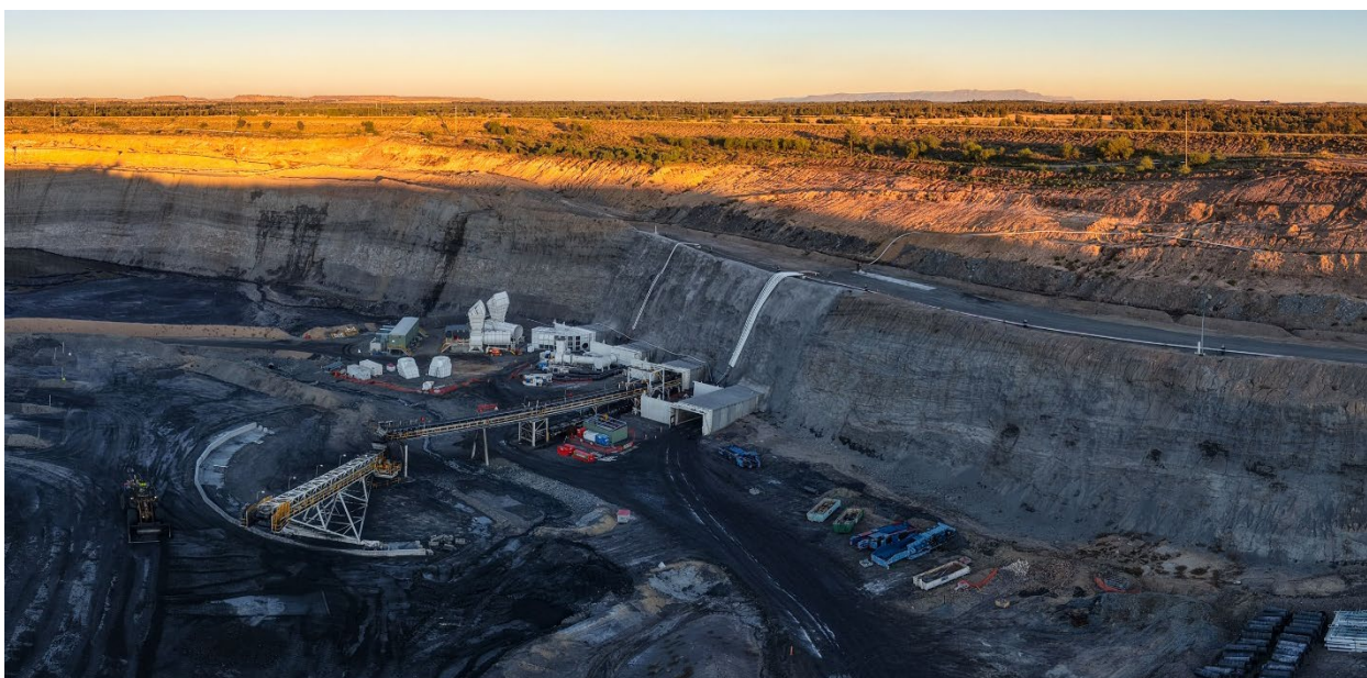
Caption: Mammoth Underground Mine – Portal and Surface ROM Infrastructure
