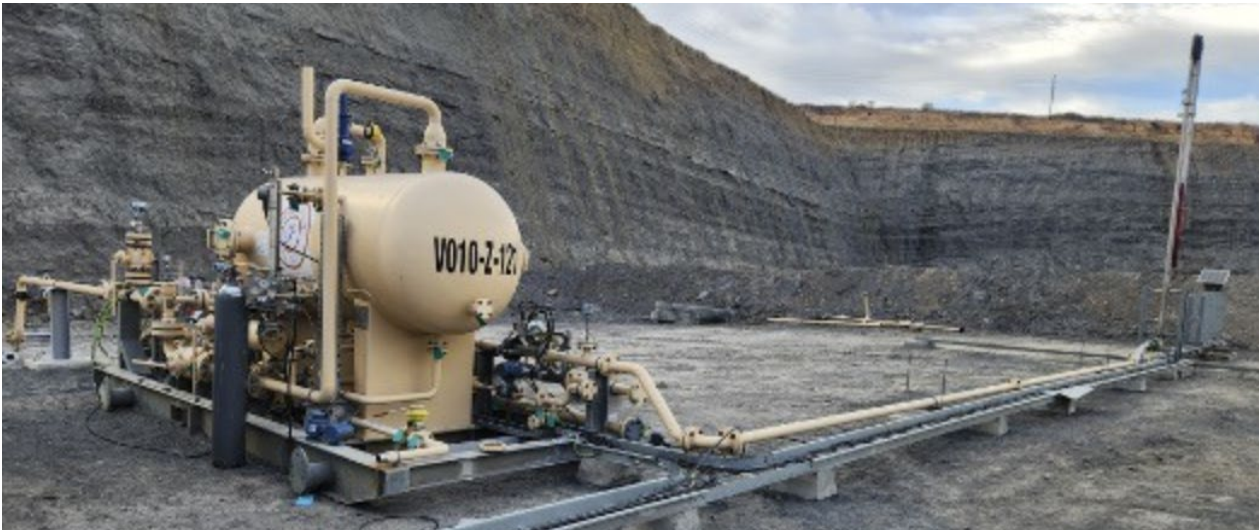
Caption: Curragh Complex, Mammoth Gas Drainage Project Infrastructure
