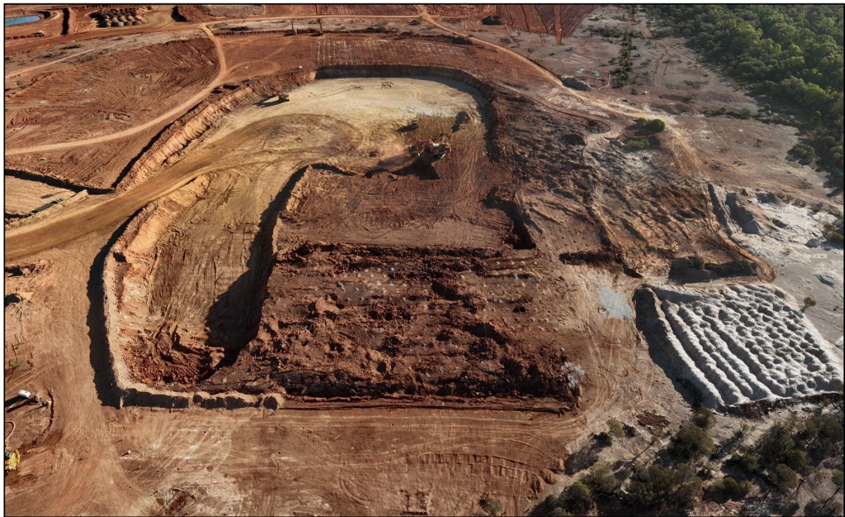
Figure 1 – Mining progressing on the first bench of the Stage 1 open pit at Crown Prince
