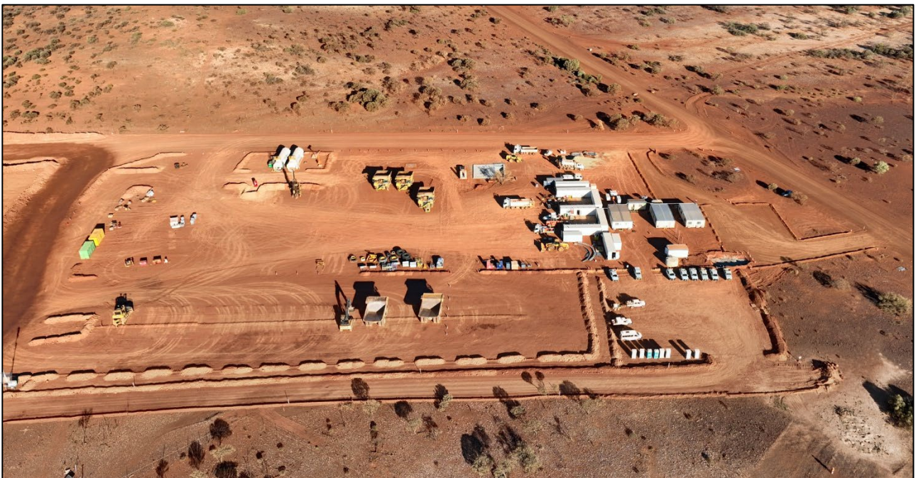
Figure 3 – Mine Office, Workshop, 'Go' Line. Construction almost complete
