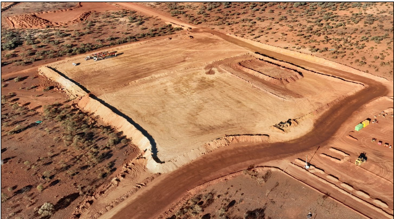
Figure 5 – Ore Stockpile being built on ROM
