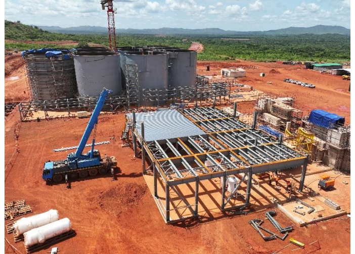
Figure 4: Grinding and CIL Tank Erection
