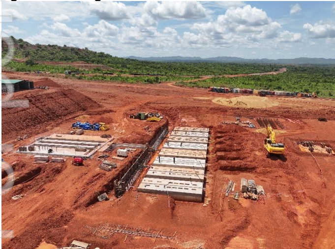
Figure 5: Power Station – Concrete Poured for 8 engine bases
