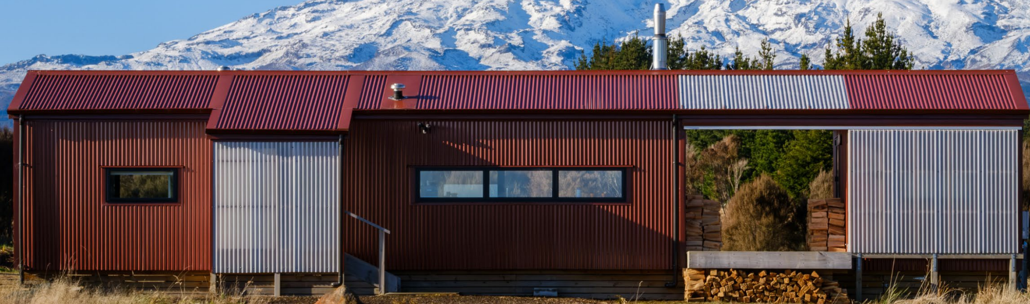
Pictured: Ruapehu Hut in Horopito, New Zealand, featuring roofing and cladding in COLORSTEEL® Scoria
