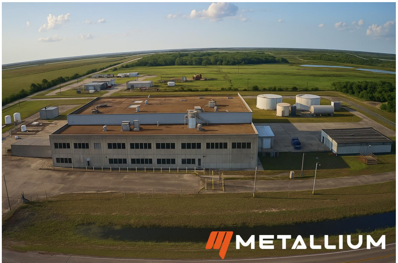
Figure 1: Metallium’s Chambers County, Texas Technology Campus – Front Entrance. Facility undergoing upgrades ahead of December 2025 commissioning
