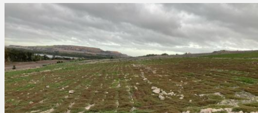
Peak Downs Rehabilitation Works
