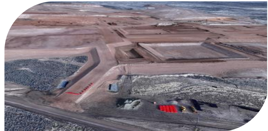
Commencement of Major Construction in May 2025
