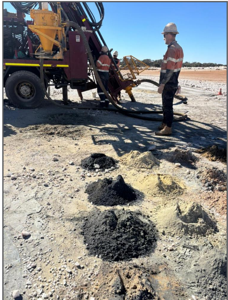
Figure 1. Aircore drilling commences at Goongarrie.
