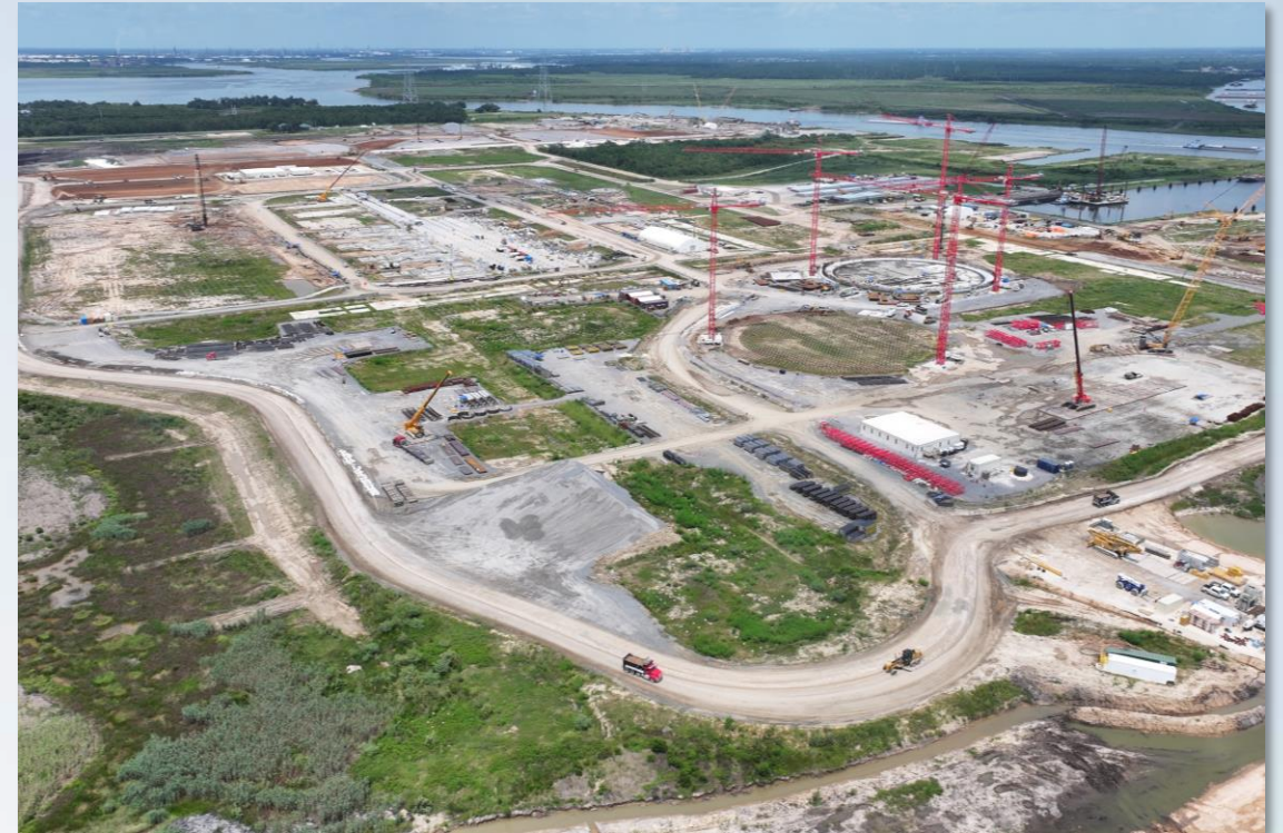
Woodside Louisiana LNG site, 7 August 2025
