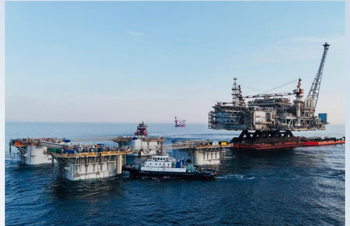
The Scarborough FPU hull and topsides were successfully connected in May 2025
