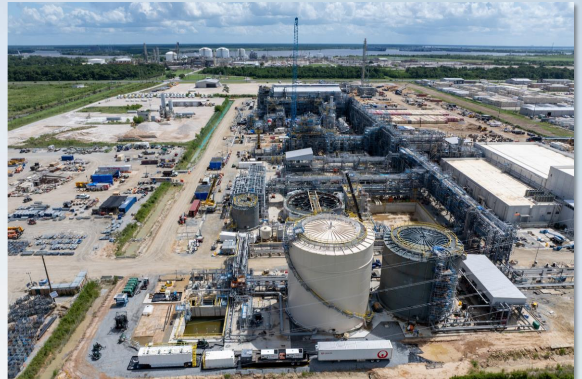
Construction of the Beaumont New Ammonia Project in Beaumont, Texas
