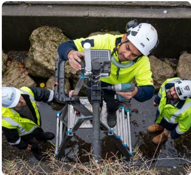
Technicians installing solar-powered sensors in Havelock North.
