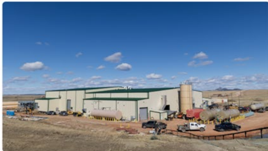
Central Processing Plant (Phase I & II)
