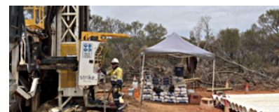
Water bore drilling
