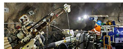
Underground infrastructure drilling
