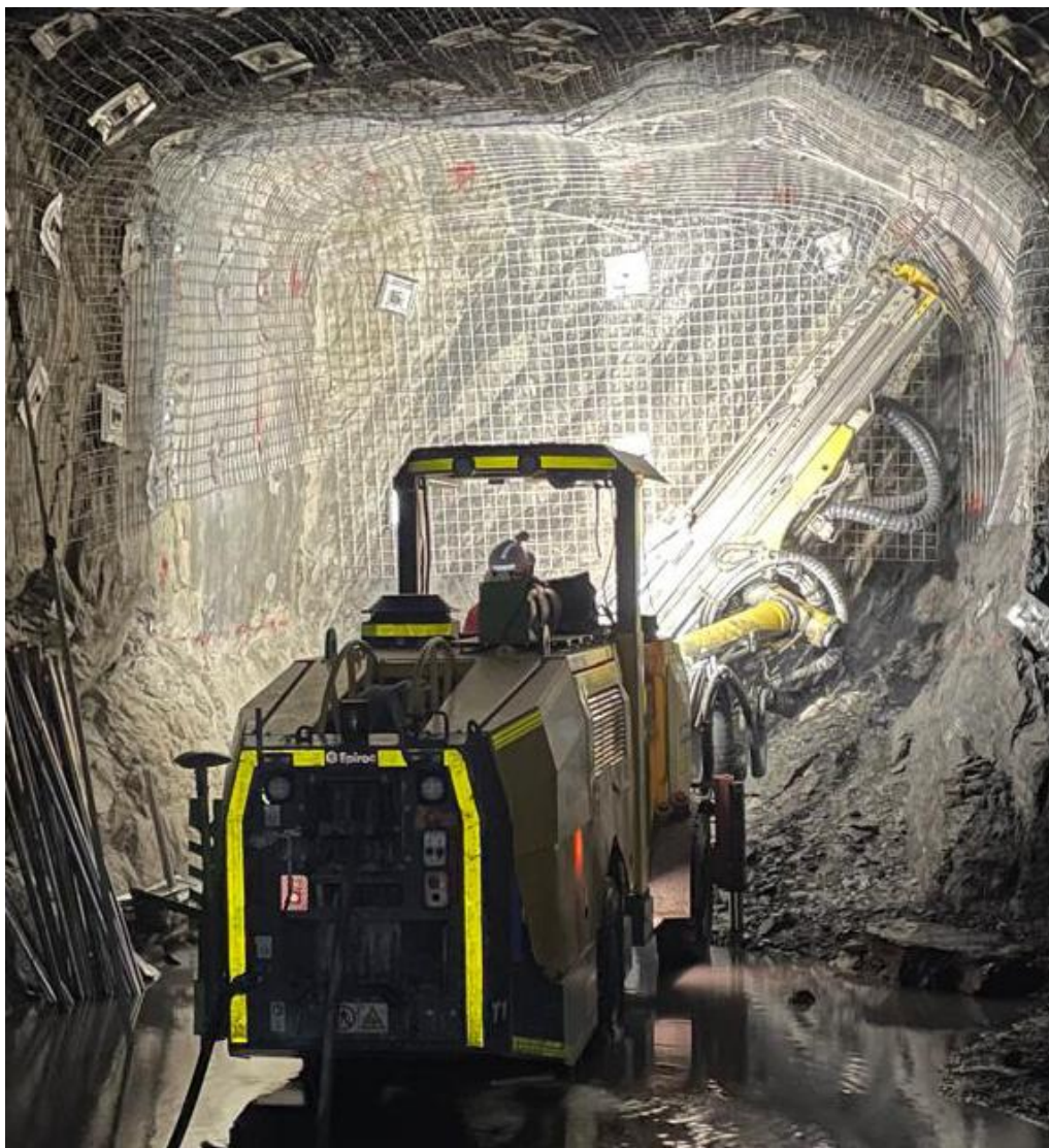
Figure 2 – Jumbo bolting drill caddy on Lady Belmore Vein.
