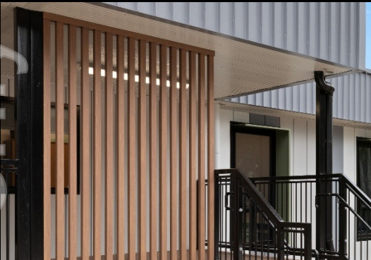
Commercial Bluescope Offices NSW
