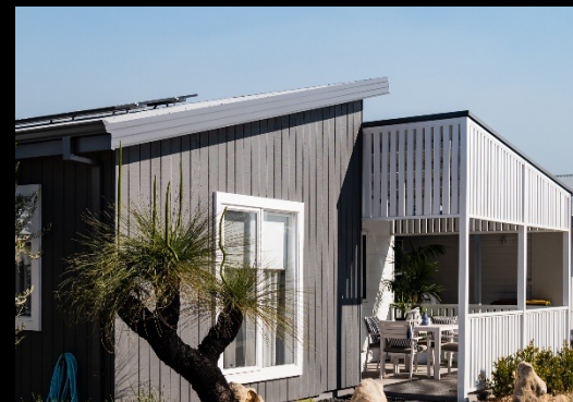
Housing Piara Waters WA
