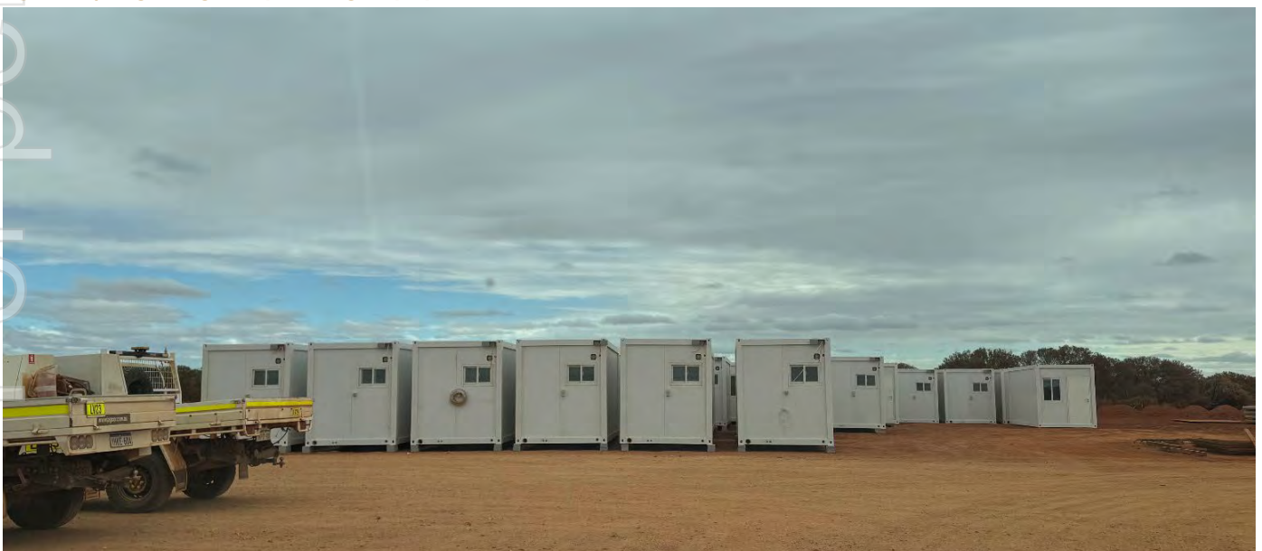
Figure 15 | Dingo Range camp buildings in preparation for installation
