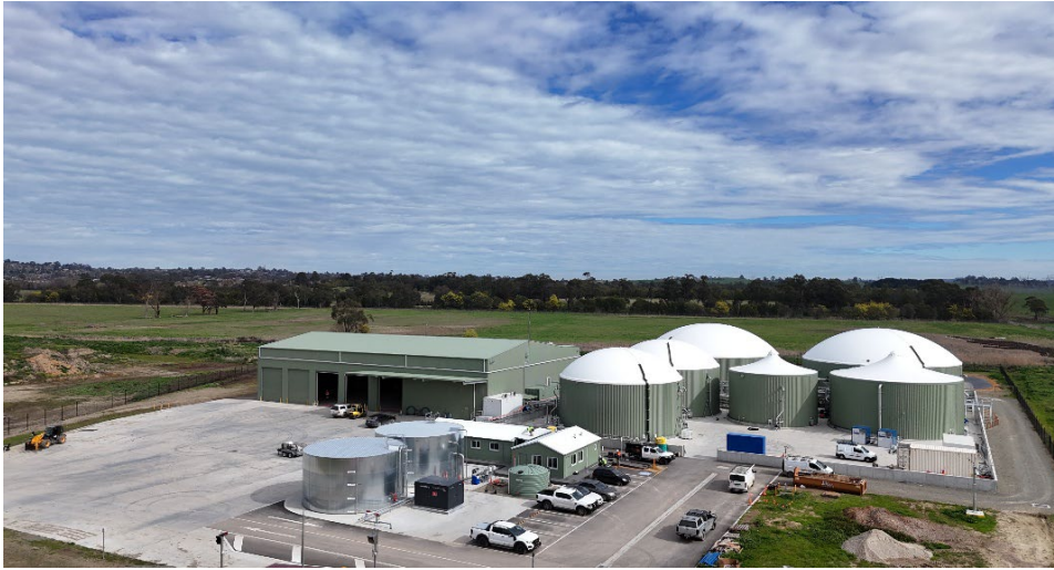
YVW Lilydale Food Waste to Energy Project
