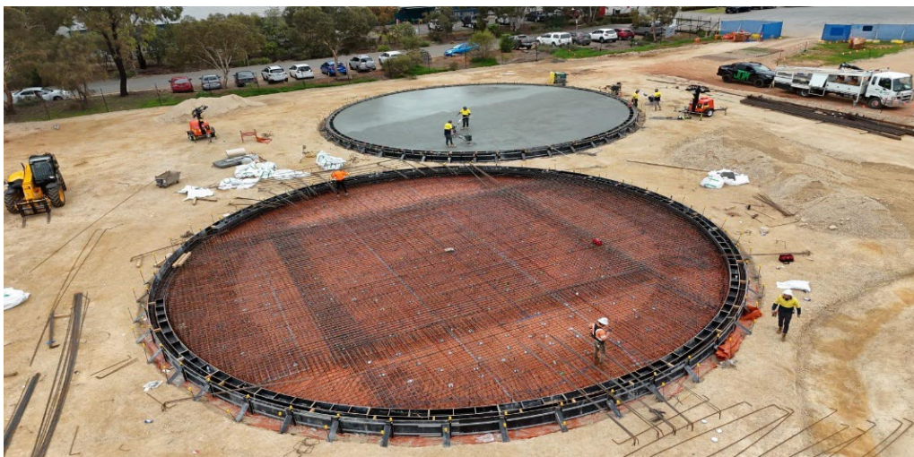
SA1 Salisbury Bioenergy construction
