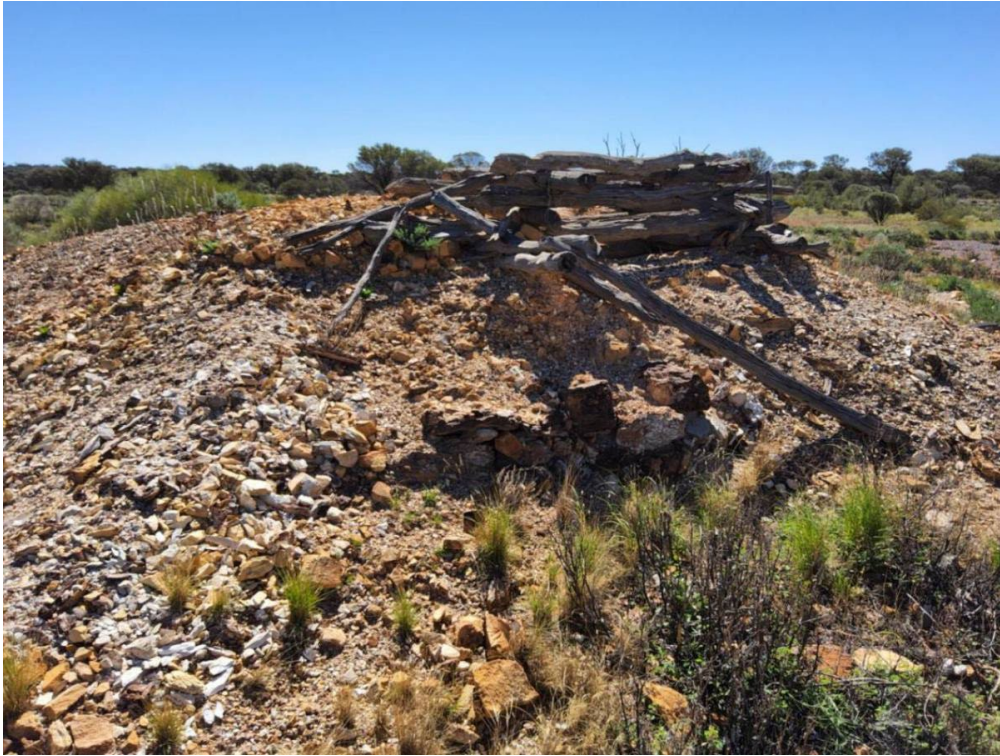
Figure 6. Leonidas — historical shallow shaft developed in weathered dolerite along a linear magnetic high. (MGA94 Z51 - 382708mE 6793453mN)
