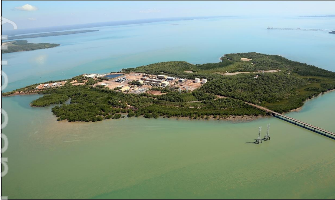
Channel Island Power Station. ~300 MW natural gas-fired power station located in Darwin
