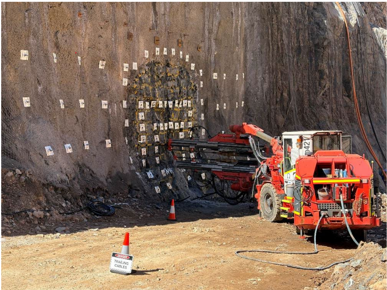
Figure 1: Majestic main decline portal, prior to firing.
