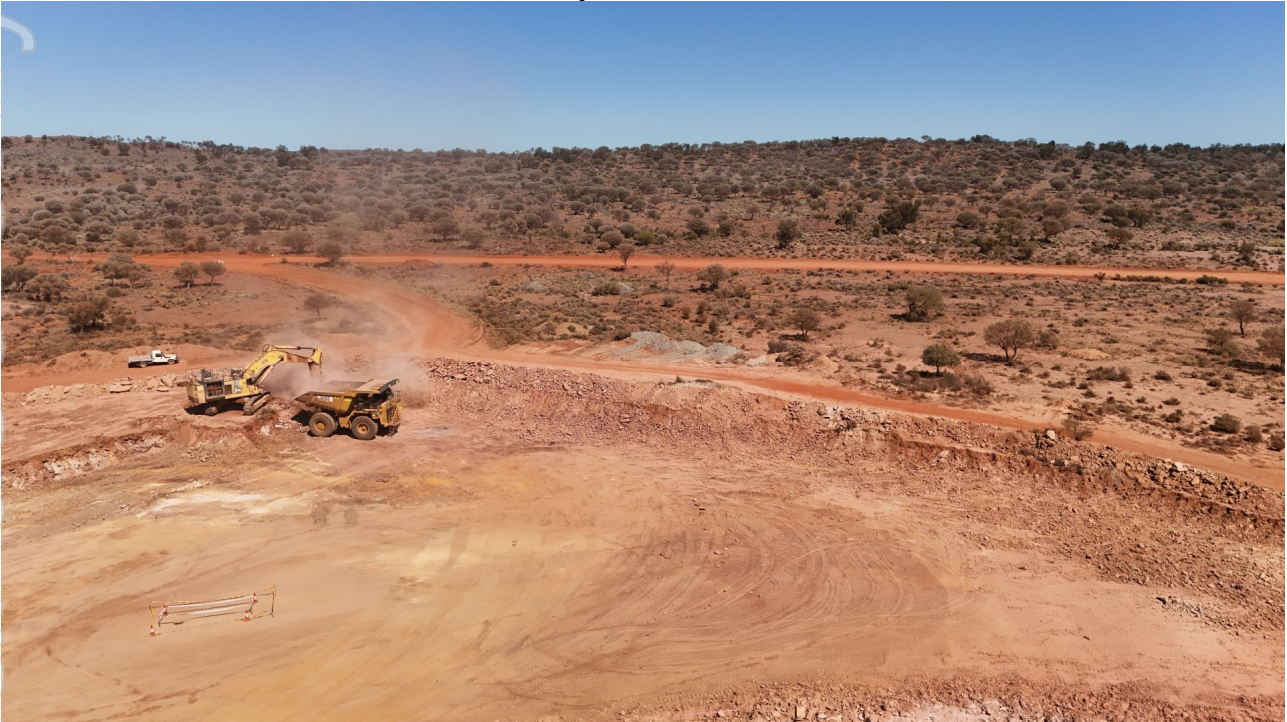
Photo 1: Neta Commencement of of Open Pit
