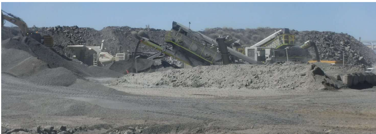
Photograph taken by Derisk during site visit, 2024.
