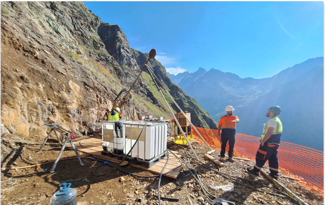
Picture Man-portable drill rig positioned on platform 2 at Zopkhito
