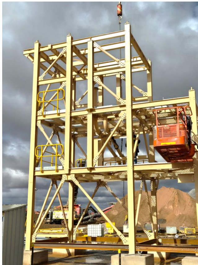
Figure 7: Installation of the gravity tower at the 1.2mtpa Lakewood processing facility
