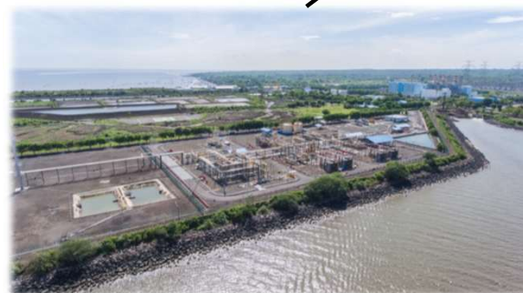
Existing Grati gas processing facility
