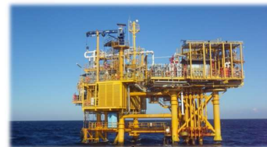
Existing Oyong pipeline to shore
