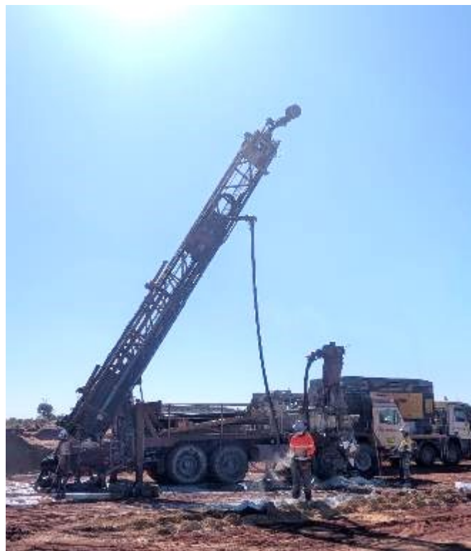
Drilling underway at the Apollo Hill Gold Project.
