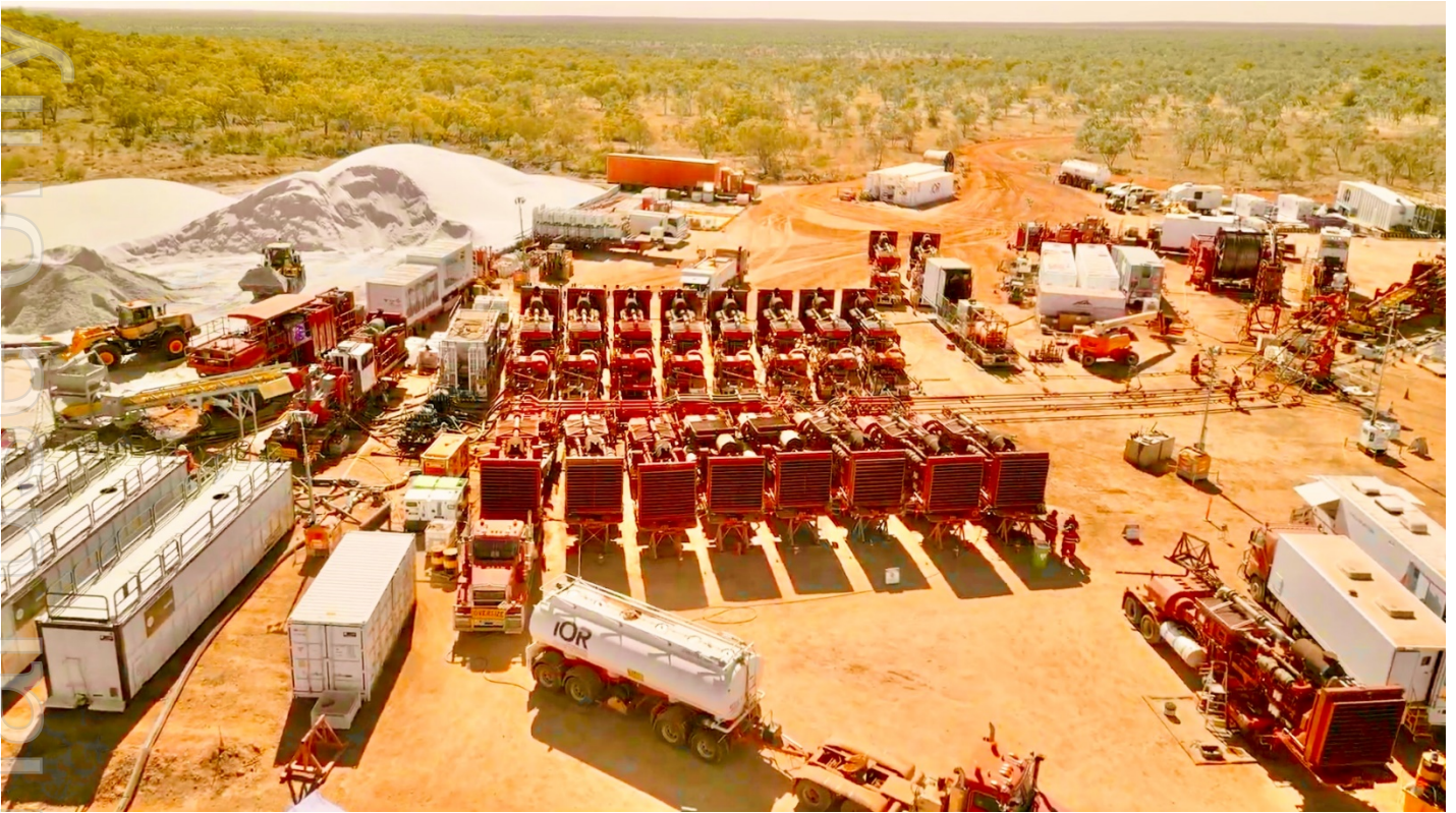
Halliburton frac spread at Carpentaria-5H
