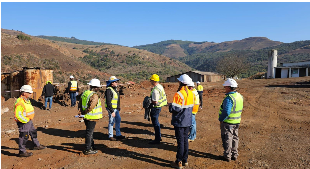
Figure 1: Site visit with the execution team and contractors August 2025
