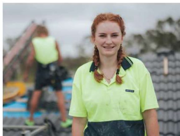
Photo: Our female roof tiling apprentice is raising the roof for other female trade apprentices
