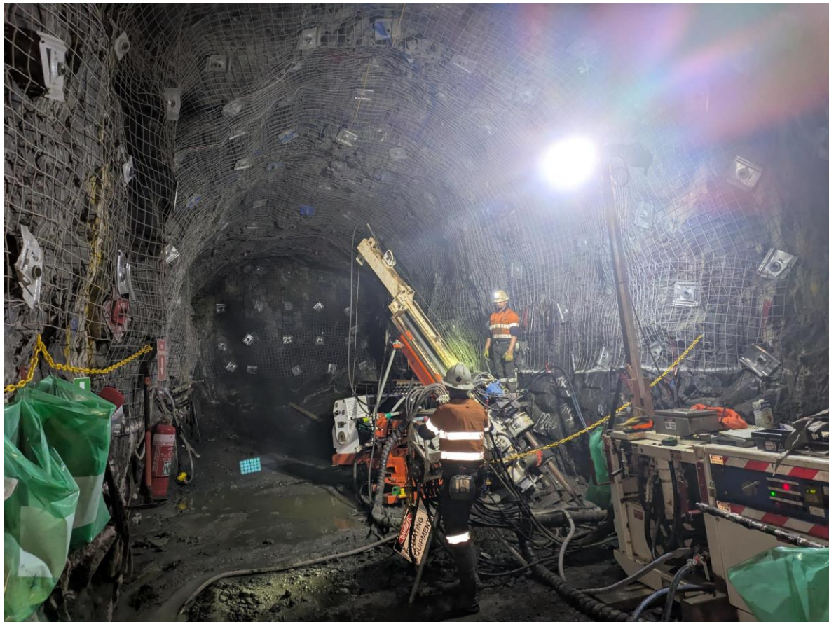
Figure 4 - Underground diamond drilling at the Fish Mine
