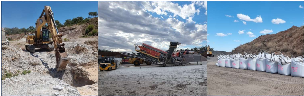
Figure 4: Left – Excavating the bulk sample from trench T7 and loading directly into a waiting truck; Middle – Sample being loaded into the crushing and screening plant in Condobolin, where the sample was crushed to -40mm and screened to separate the -7mm fines; Right – Sample awaiting transport after being loaded into bulk bags for transport to TOMRA Ore Sorting Solutions, Sydney for full-scale ore sorting testwork before downstream concentrating in pilot-scale processing plants at ALS Perth and then ALS Burnie.
