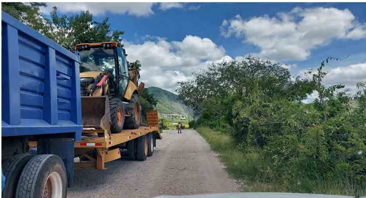
Road infrastructure machinery mobilized. Work commenced.
