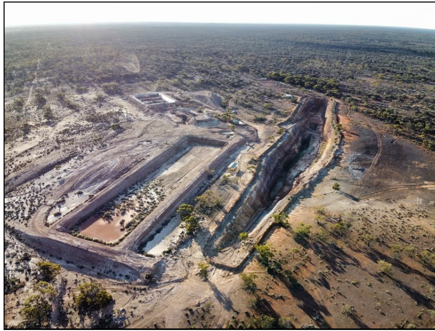
Figure 4: Drone photo of Zelica Project looking NNW showing pre-stripped open pit (approx. 300m long and 10-25m deep) and pre-constructed vat leach ponds (pic taken August 2025)
