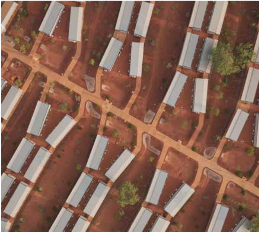
Mine Accommodation area
