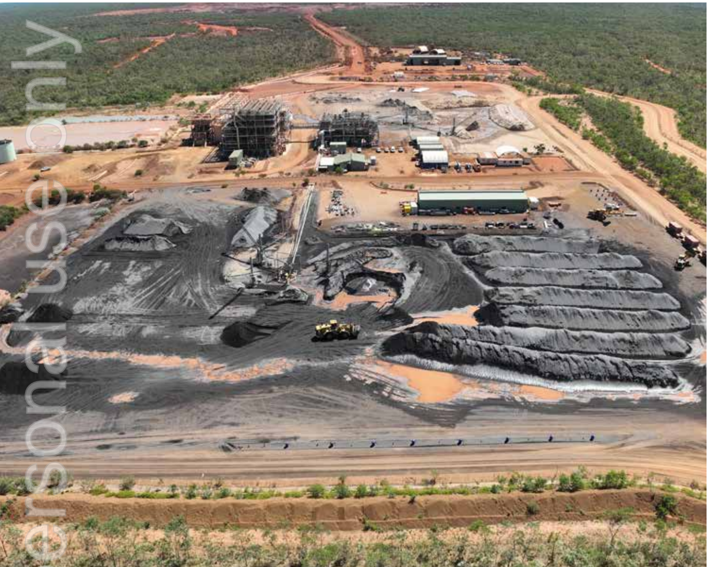
Thunderbird Process Plant and stockpile area
